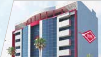
Laying the foundation stone for the new headquarters SUNU Assurances companies in Burkina Faso
